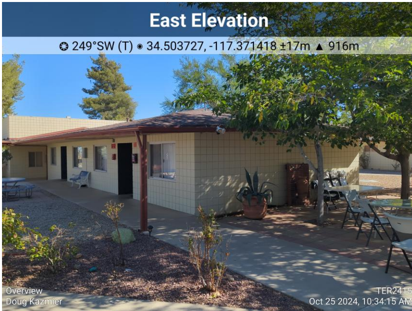
Photo 6: St. John of God Building (View West).
