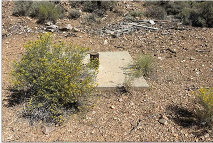
Photo 13. Feat-4 consisting of ventilation shaft. View towards north.
