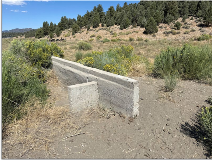
Photo 3. Feat-3 consisting of wall and foundation. View towards northwest.
