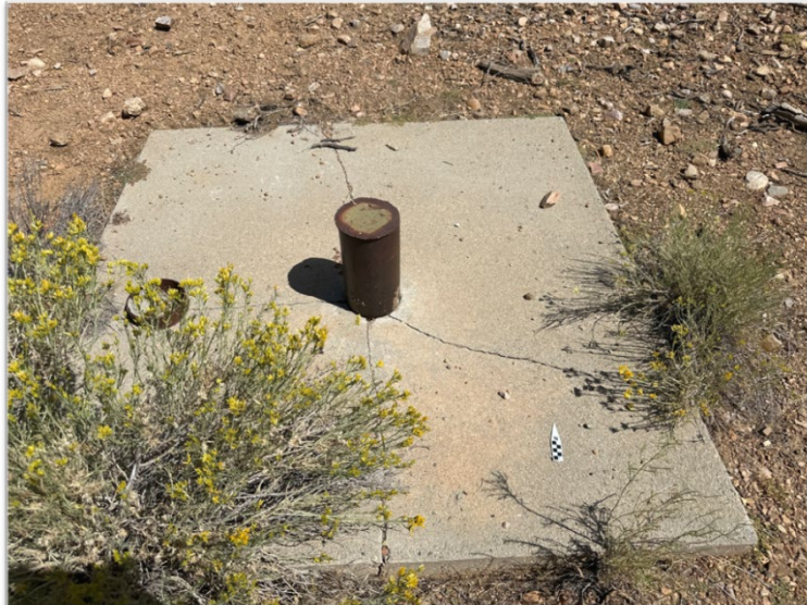
Photo 14. Feat-4 consisting of ventilation shaft. Detail view.
