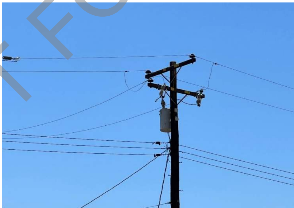
Photograph 10: View of pole-mounted transformer in the vicinity to the south of the site.
