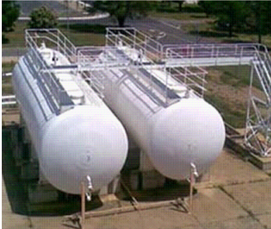
STANDARD TANK TOP PLATFORM AND LADDER
